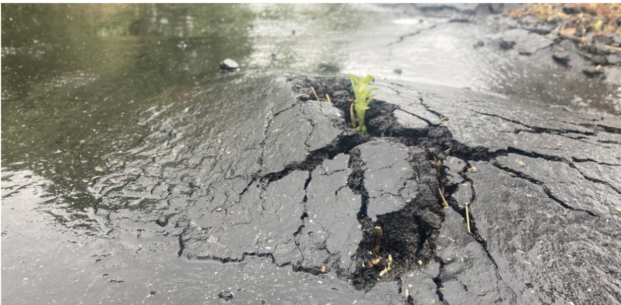
A shoot from an underground willow root is seen breaking through a recently paved asphalt walkway.
